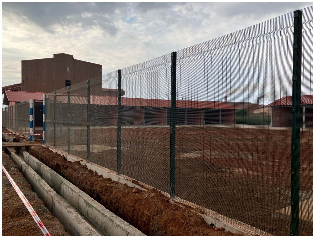
Figure 8-6 The hazardous waste facility in Kamsar (under construction)
